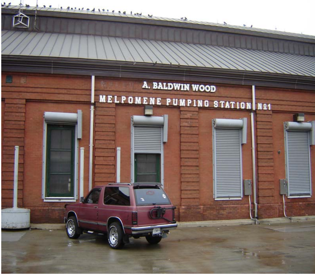
OP #1 Melpomene Pump Station #1
