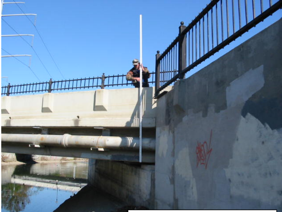
Low Chord Northline Street East -3.288 feet NAVD88 2004.65 Field Book 060852
