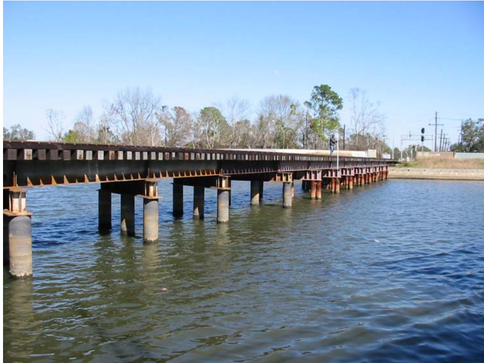
Low Chord Railroad Bridge by OP #6 5.46 feet NAVD88 2004.65 Field Book 060850
