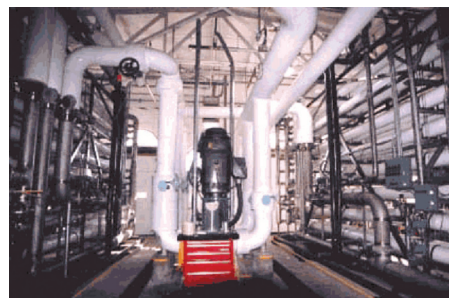
(Left photograph) A desalination plant for the City of Cape May, New Jersey, was built inside the brick building of the former Cape May Water Works. (Right photograph) The automated desalination plant can produce from 750,000 to 2 million gallons of water per day. (Photos: Jennifer Kopp, courtesy of CapeMay.com)
