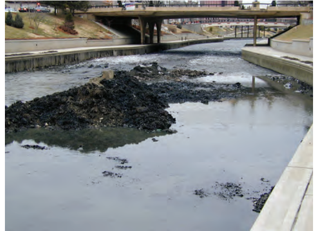
Figure 33. Sediment accumulation in Plaza pool, upstream from site 10, being prepared for removal, January 2000.
