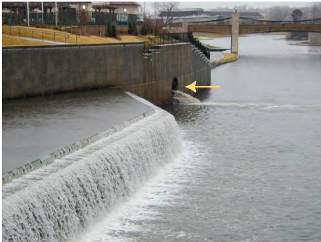
Figure 3. Flow over weir from Plaza pool (above site 10) into Volker pool below (above site 11) following storm event and storm sewer discharge into Brush Creek (marked with arrow).
