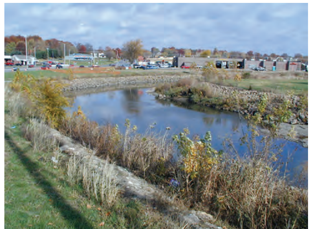
Channelized reach of Indian Creek upstream from site 6.
