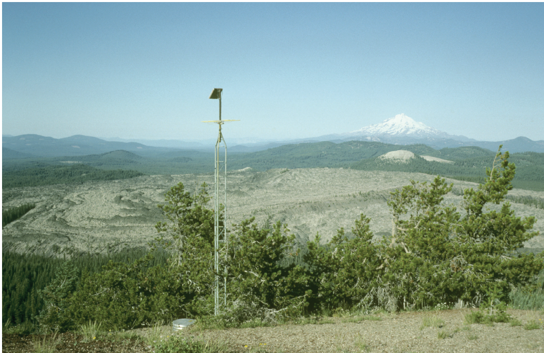
Figure 18. This seismometer installation on the upper west side of Medicine Lake volcano at Little Mount Hoffman is one of only two seismic instruments that are located on the volcano. View is southwest across the Little Glass Mountain flow that erupted about 1,000 years ago. Mount Shasta is on the horizon.
