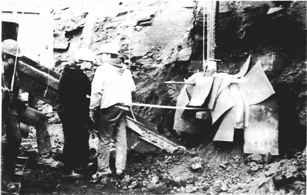
Figure 1.—Inert gas shroud enclosure of auger hole collar. Note small-diameter pipe used for collar measurements.
