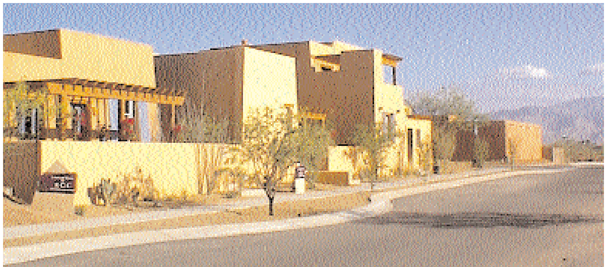
Civano, Arizona. Social edge streetscape. Shows the variety achieved in the street front by paying attention to design elements. All garages are in back alleys, and therefore there are voids in the public street front. This street front is a good example of a strong social edge. All houses have porches, and the design elements from the sidewalk to the front door-steps, porches, trellises, walls, etc., have been given careful consideration to create zones of varying privacy. This invites interaction with neighbors
