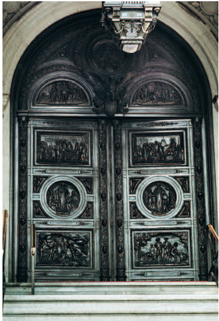
Doors to the Capitol
