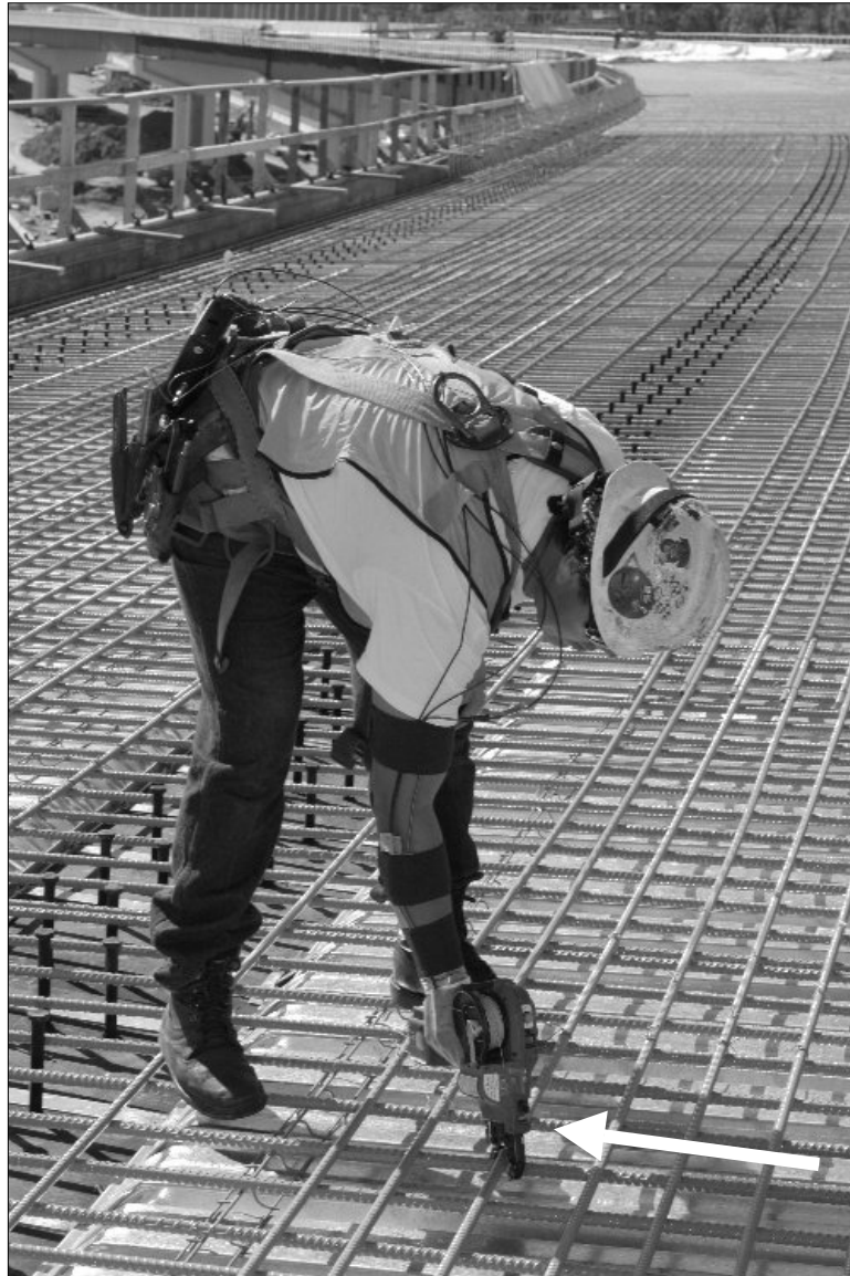
Figure 4 Rebar tying using MAX-USA RB392 battery powered rebar tier
