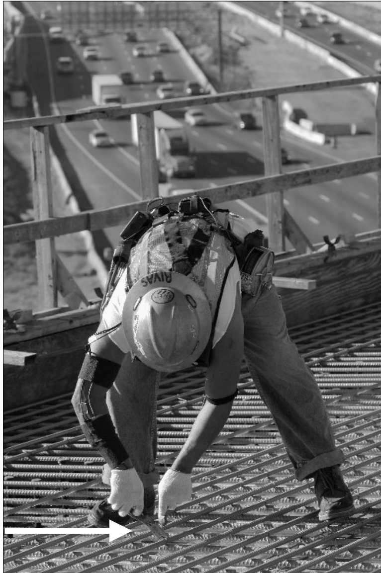
Figure 3 Rebar tying using pliers and tie-wire
