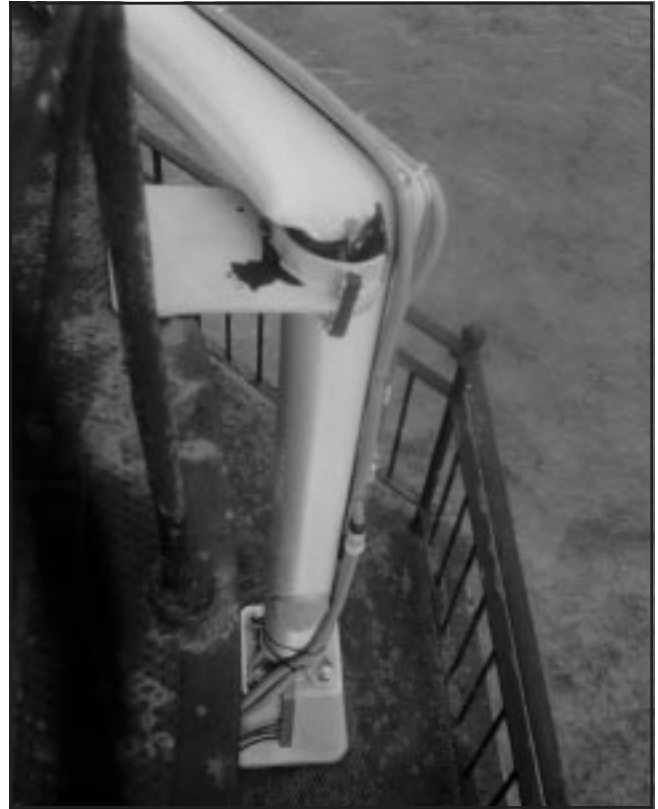
Fowey Rocks trolley mast bent 90° by Hurricane Andrew.
