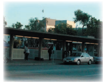
Shelters such as these, with high roofs and no side walls, provide little protection from wind or rain, and should be avoided. [Lake Merritt]
