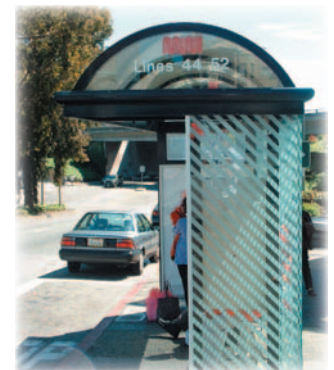
The best bus shelters provide protection from wind and rain, while still allowing passengers a clear view of oncoming vehicles. [Glen Park]
