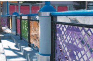
Art can humanize an environment, forge strong links with the community, and make station areas more attractive for pedestrians and waiting bus passengers. [16th Street/Mission]
