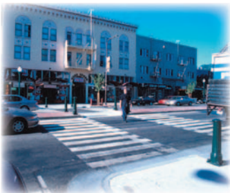
Median refuges and corner bulbouts reduce crossing distances for pedestrians, and help to slow traffic speeds. [Downtown Berkeley]
