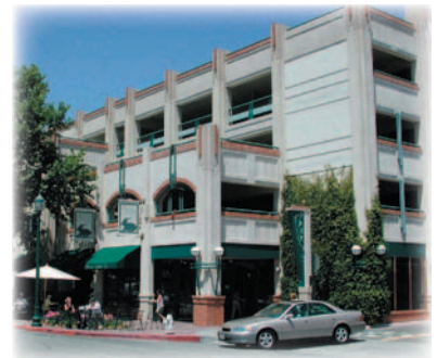
Active uses, such as retail or housing with windows facing the street, can wrap the first floor of a parking garage. They help provide natural surveillance and an interesting, attractive pedestrian environment. [Walnut Creek]
