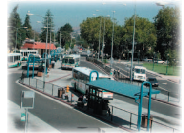
While there should be a presumption against off-street bus transfer centers, they are sometimes necessary to cater for “pulse” scheduling on infrequent routes, and ease timed transfers. [Hayward]
