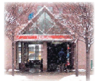
Dual-side portals minimize walking distances to nearby destinations. By orienting passengers towards their destinations as they emerge from the station, they eliminate backtracking, and also ensure that the station is visible from multiple directions. [Kendall Square, Boston]
