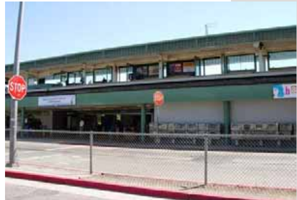
The station entrance is located on the east side of the BART property with a wide concrete apron.
