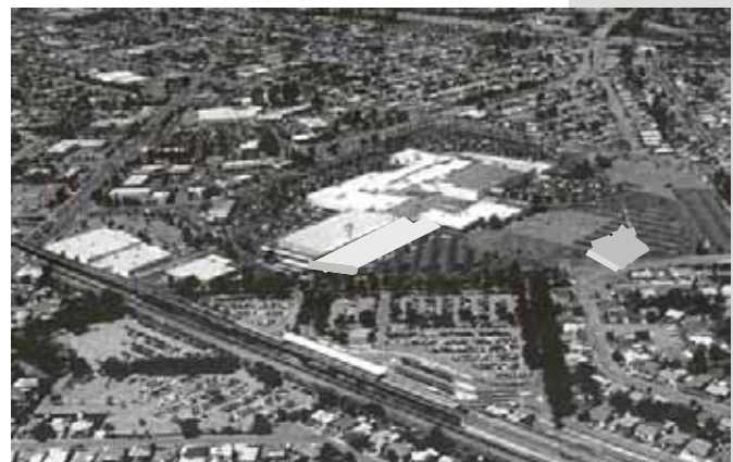
View looking over the BART Station, with Bayfair Mall, the Gateway area and East 14 th Street Corridor. Parking lots dominate the immediate area surrounding the Station, providing opportunities for infill development.
