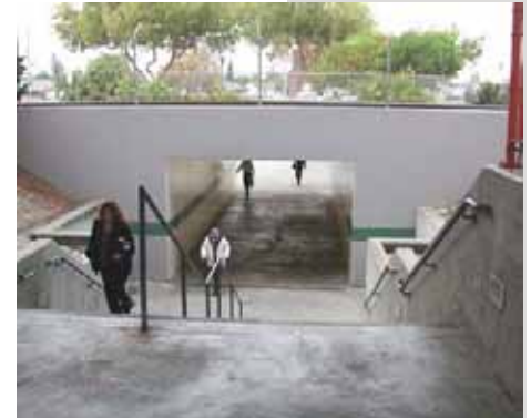
The underpass leading from the west lot to the eastern station entrance.
