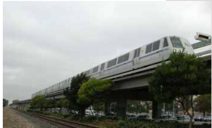
BART's Dublin/Pleasanton and Fremont lines converge at Bay Fair Station, making transfers possible. In the future, Silicon Valley trains will also stop at Bay Fair.
