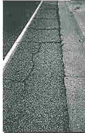
Pavement/Gutter Pan Seam (e.g., uneven, deteriorating)
