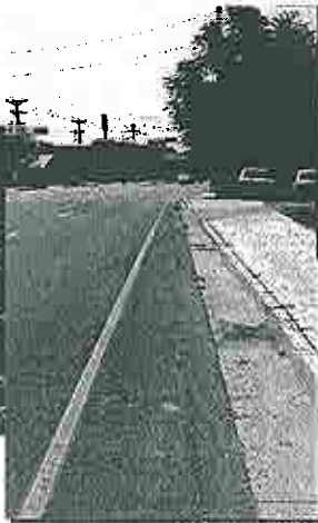
Inadequate Bike Lane Width
