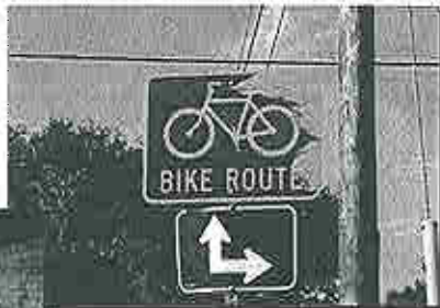
Poor Condition of Signing
