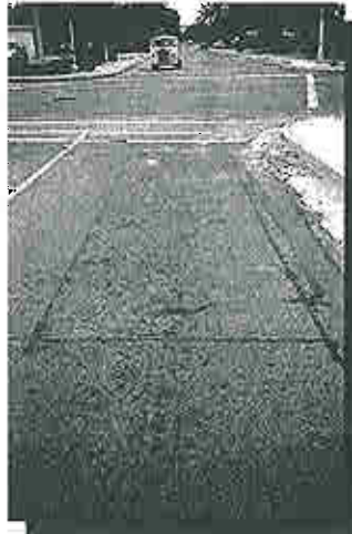
Loop Detectors not Sensitive Enough to Detect Bicycles
