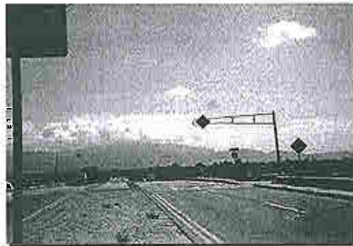
Trail crossing at a major street.
