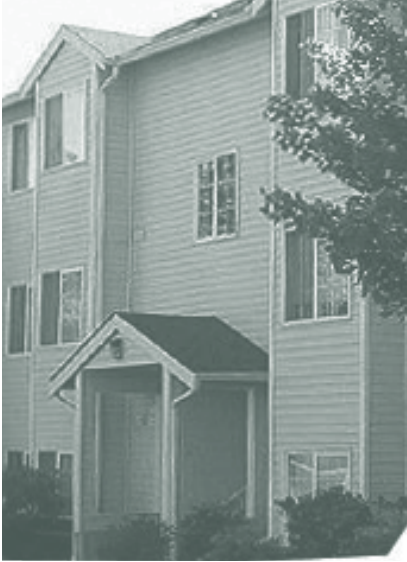
R.I.S.E. transitional living house
