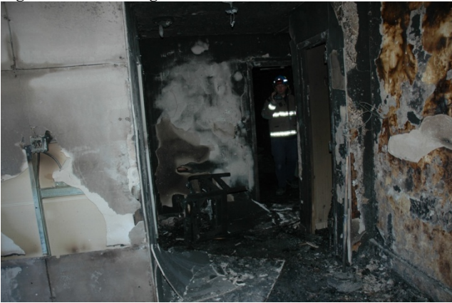
Figure 9.5-57. 3E apartment entrance from living room
