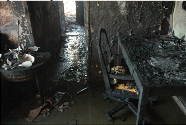
Figure 9.5-21. Living room to bedroom hallway
