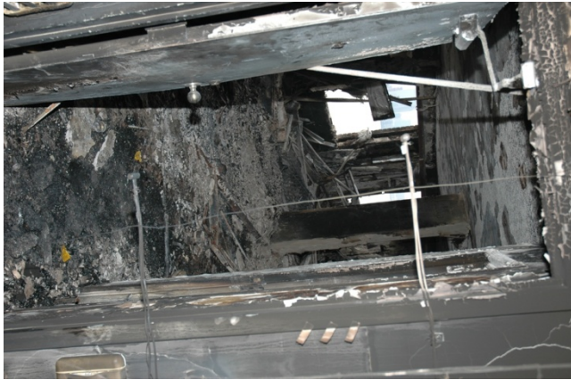
Figure 9.5-1. 7G apartment entrance
