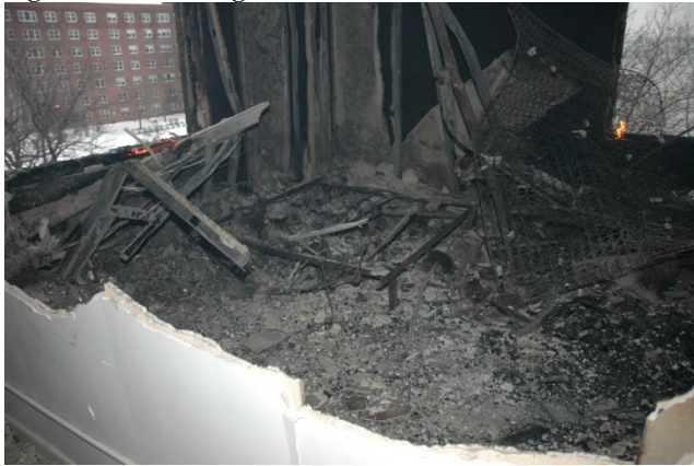
Figure 9.5-27. Bedroom windows from adjacent bedroom
