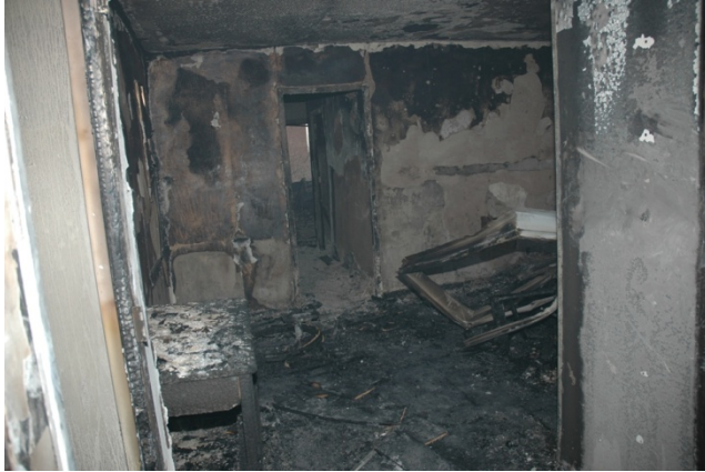
Figure 9.5-25. Living room from entrance
