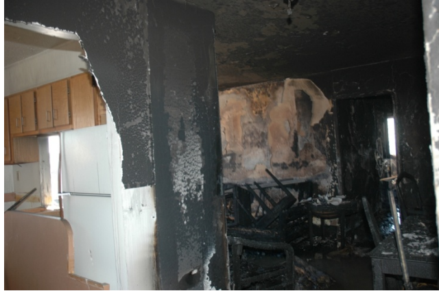
Figure 9.5-20. Living room from entrance
