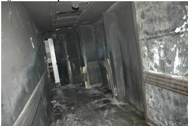
Figure 9.5-3. Down the corridor toward apartment 7K
