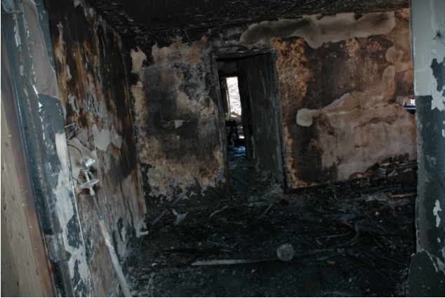
Figure 9.5-55. Living room from entrance
