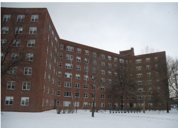
Figure 1.2-4. Rear of structure (Side C)
