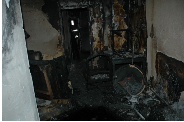
Figure 9.5-32. Living room from entrance
