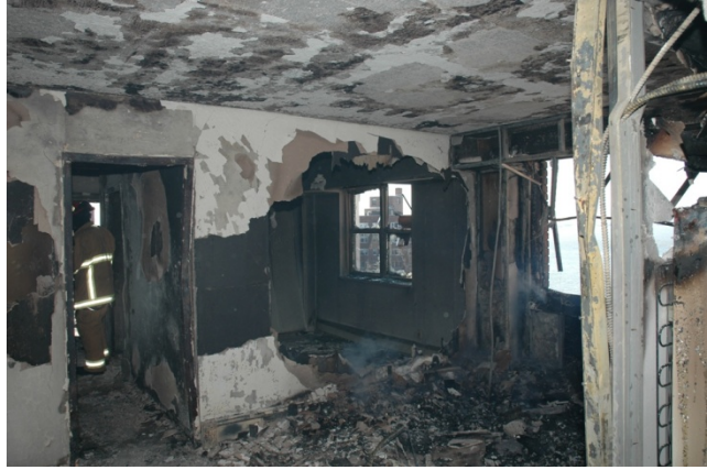
Figure 9.5-8. Living room from entrance
