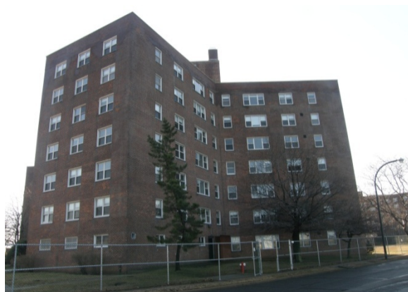
Figure 1.2-5. Right side of structure (Side D)
