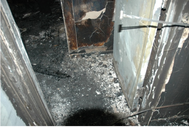
Figure 9.5-31. 5K apartment entrance
