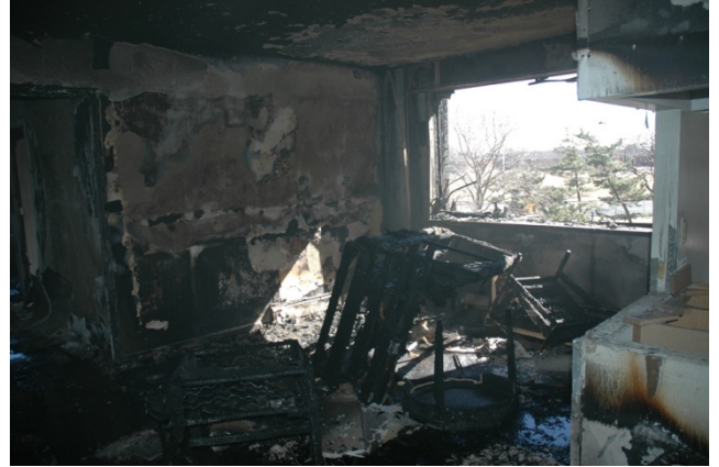
Figure 9.5-50. Living room from entrance
