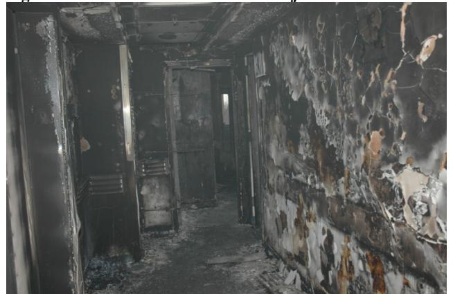
Figure 9.5-30. 5E apartment entrance from the corridor
