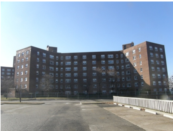
Figure 1.2-2. Front of structure (Side A)
