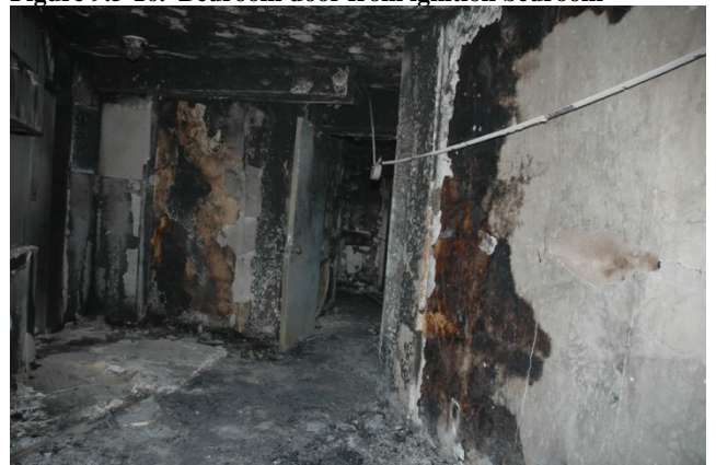
Figure 9.5-18. 7A apartment entrance from living room
