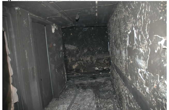
Figure 9.5-73. Down the corridor from 3K apartment entrance
