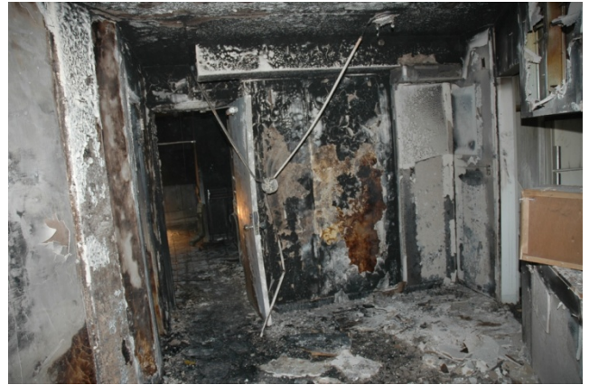
Figure 9.5-2. To the corridor from the living room
