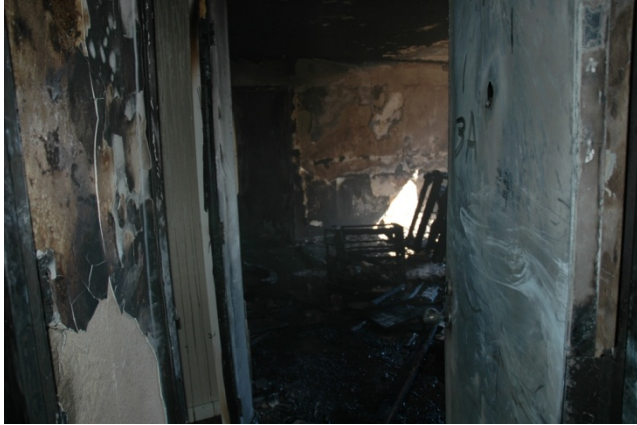
Figure 9.5-49. 3A apartment entrance
