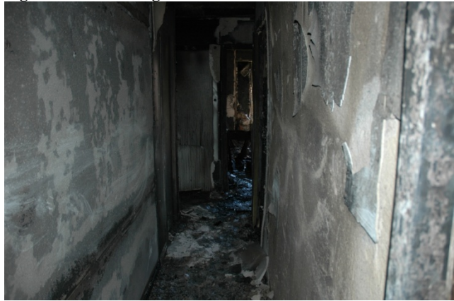
Figure 9.5-58. Living room to bedroom hallway
