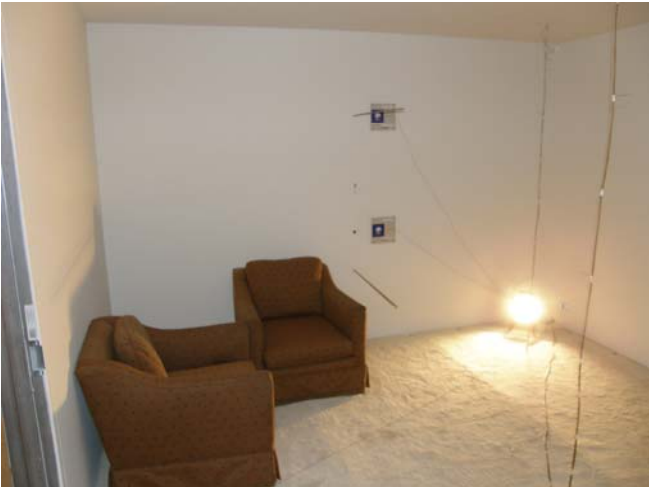
Figure 4.1.3-5. Gas sampling probe installation on south wall of living room.
