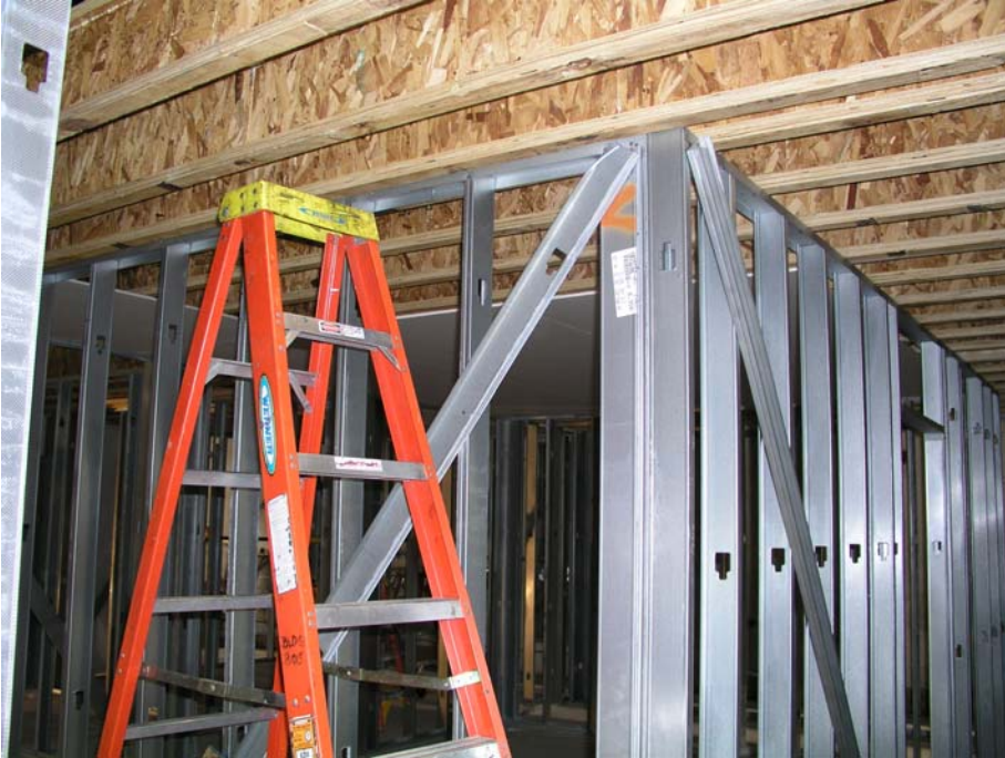
Figure 4.1.1-3. Ceiling supports for experimental structure.
