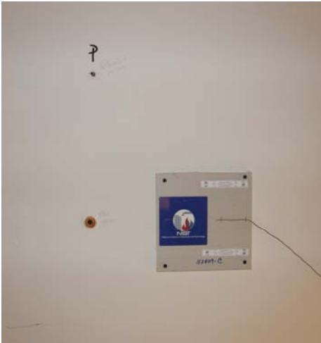
Figure 4.1.3-4. Wall mounted thermocouples, heat flux sensor, and differential pressure sampling port.
