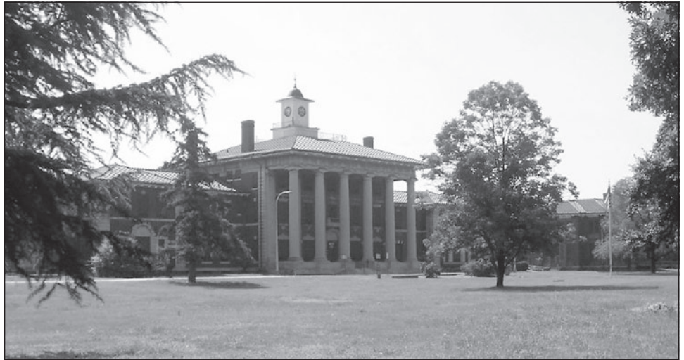
Figure 6: The Administration Building on the West Campus of St. Elizabeths
