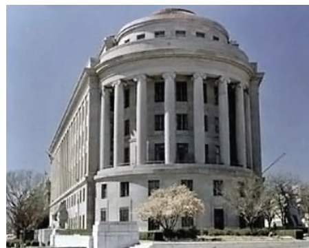
Many buildings in the Nation's capital are covered with limestone. The Apex Building/Federal Trade Commission has an upper exterior of Indiana limestone. (USGS photograph)
