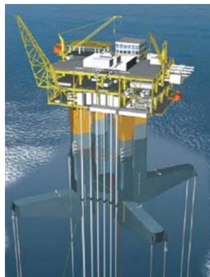
Below the surface of the Marco Polo TLP. Graphic courtesy of MODEC International.
