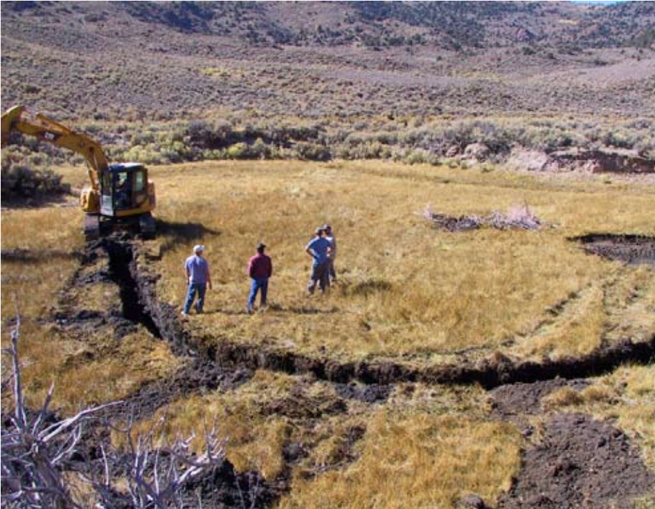
Upper photo: Construction of Horseshoe Pond begins. Lower photo: Horseshoe Pond after completion.
