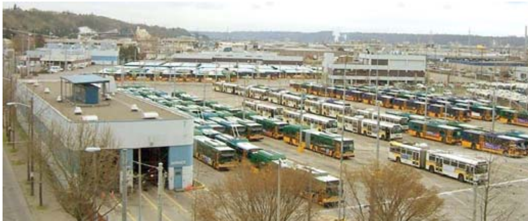
Figure 14. Bus Parking at Atlantic Base with Central Base Depot in Background
