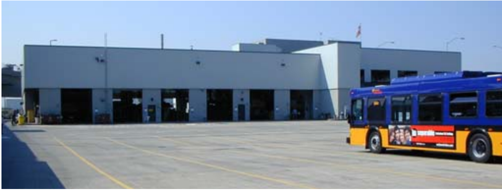
Figure 12. Ryerson Base Maintenance and Office Building
