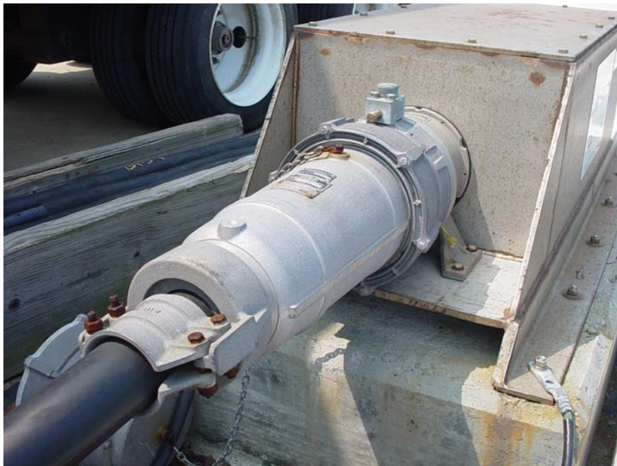
Figure 13-2. Close-Up of Electrical Connection Outlet Assembly
