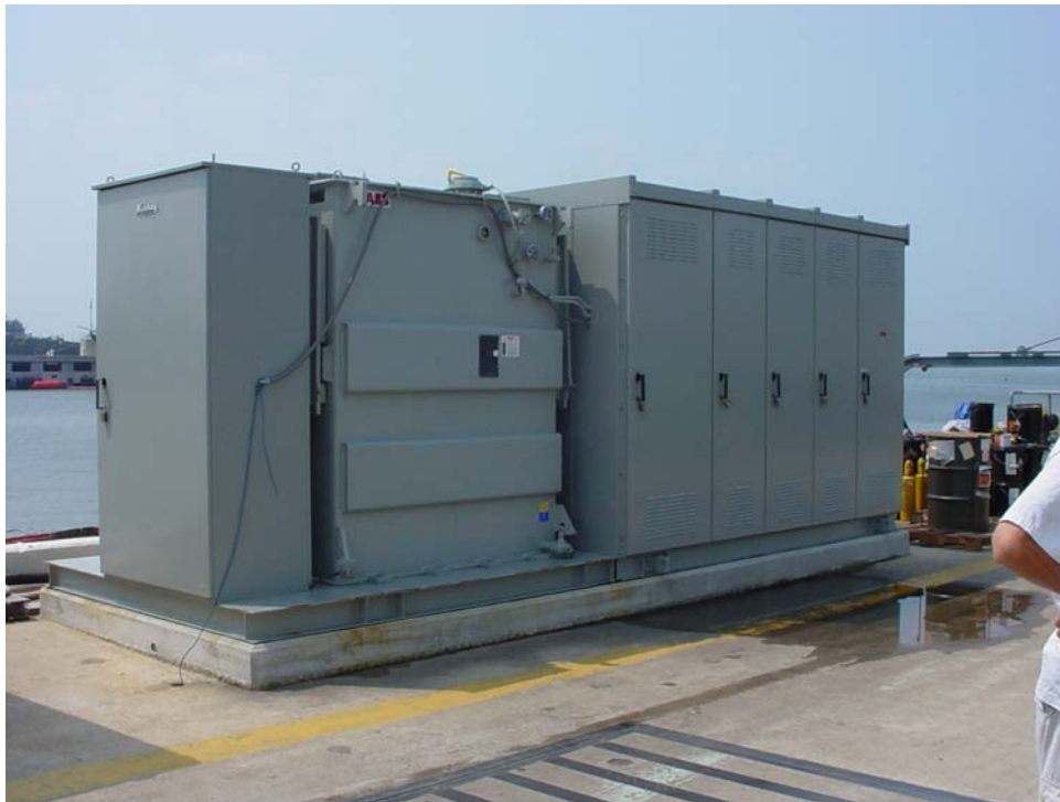
Figure 13-4. Skid-Mounted Substation
