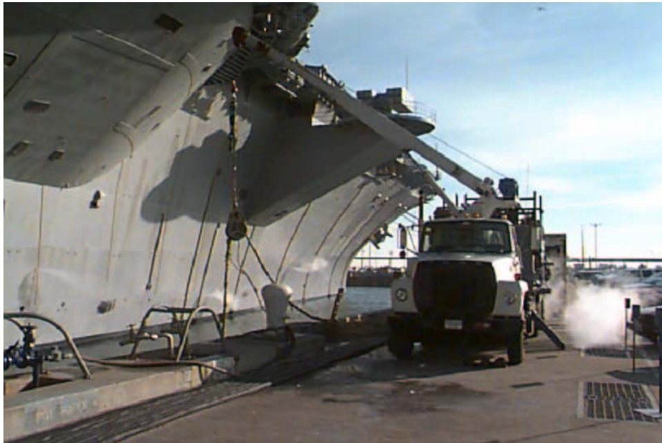
Figure 13-17. Cable Being Reeled by a Boom Truck.
