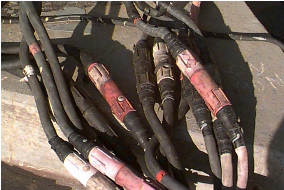
Figure 13-11. 480 Volt Shore-Cable to Ship-Cable with Single-Pole Connection
