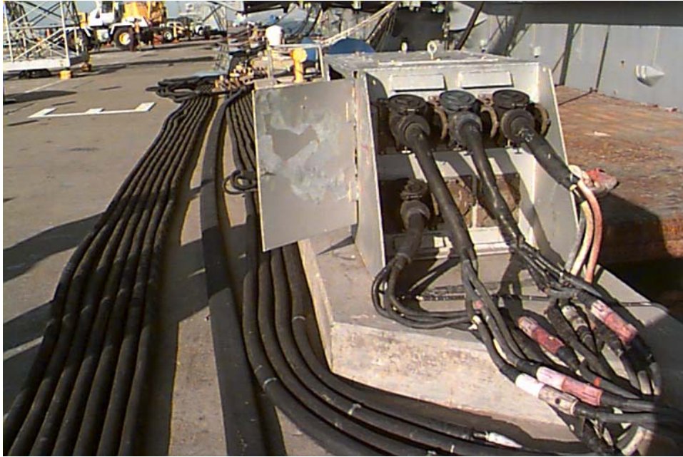
Figure 13-13. 480 Volt Shore-Cable to Ship-Cable Splice Connection in Place
