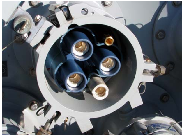
Figure 13-9. 4.16 kV Pier Electrical Outlet Assembly and Outlets – Newer Designs
