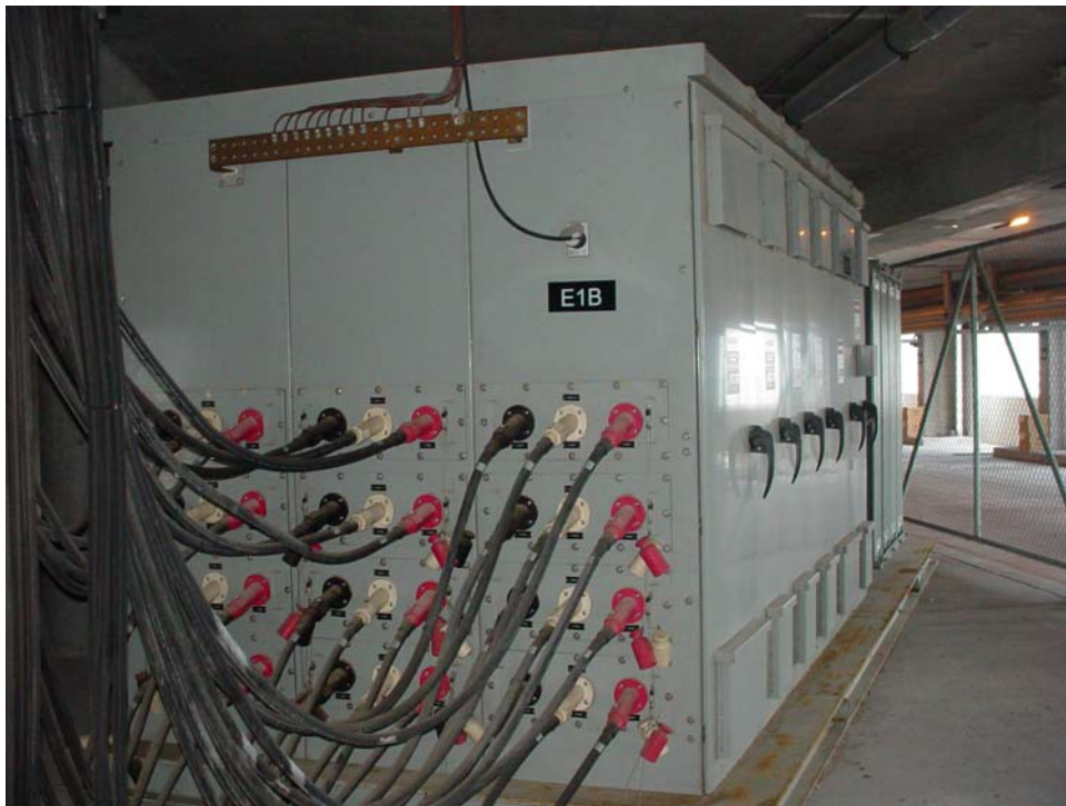
Figure 13-6. Newer Double-Deck Pier Switchgear
