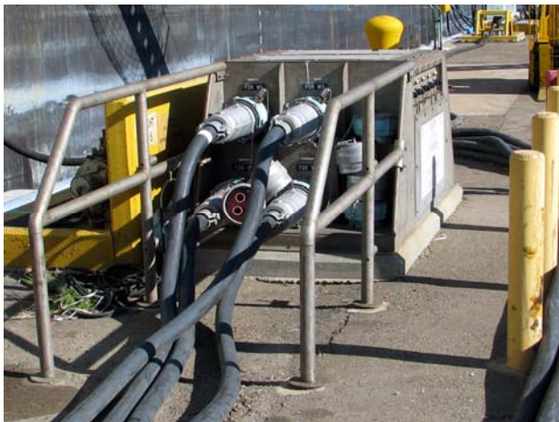
Figure 13-9. 4.16 kV Pier Electrical Outlet Assembly and Outlets – Newer Designs
