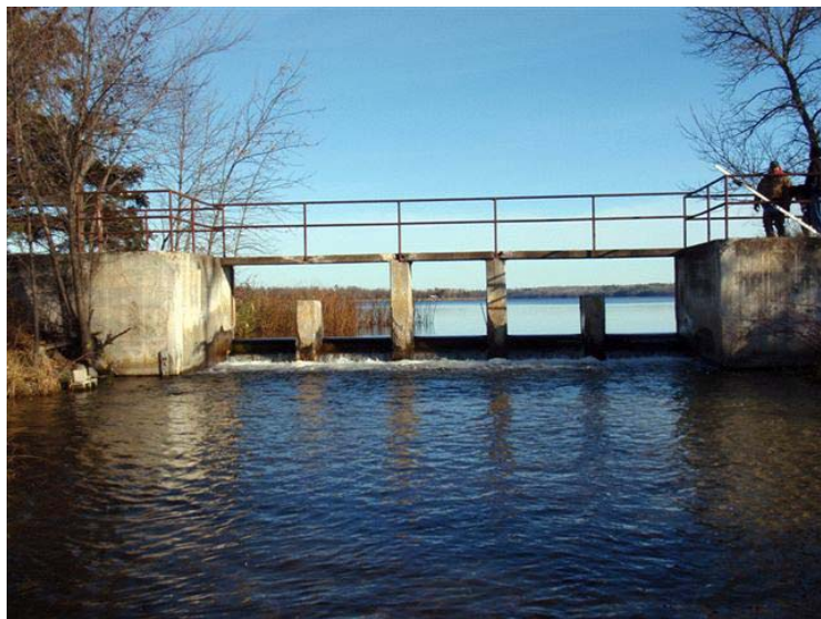
(above) Dam at Many Point Lake on the White Earth Reservation before fish passage improvement; (below) Rock and boulders were placed in the river below the dam to elevate the bottom and create a 4% slope which allows fish to pass over the dam.
