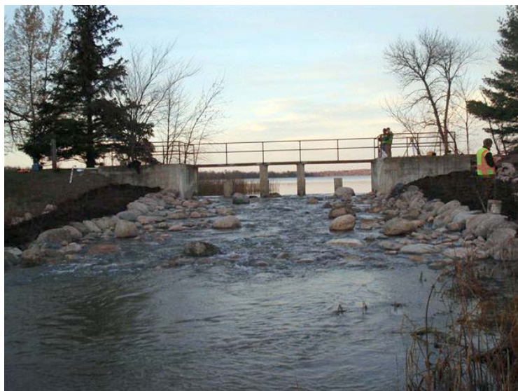
(above) Dam at Many Point Lake on the White Earth Reservation before fish passage improvement; (below) Rock and boulders were placed in the river below the dam to elevate the bottom and create a 4% slope which allows fish to pass over the dam.
