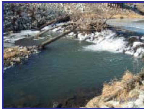
A water control weir on Seven Mile Creek in Southwest Iowa (above) was modified into a riffle approach (below) to provide uninhibited fish passage.
