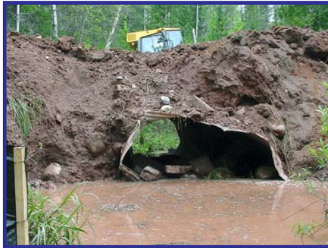
This damaged culvert (above) was replaced (below) on the Bark River providing brook trout with uninhibited access to 0.7 miles of prime spawning and nursery habitat.
