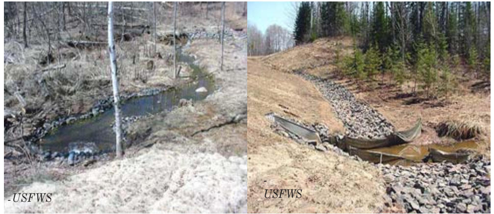
Creation of meandering streams with stabilized banks create ideal brook trout spawning habitat on Red Cliff Creek. To preserve restored habitat, erosion control measures must be placed at road crossings.
