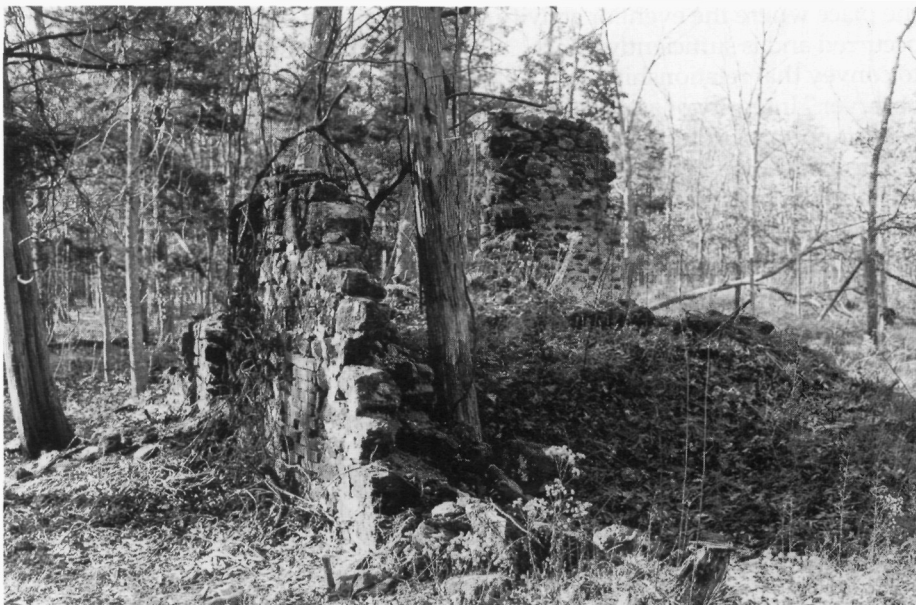
Figure 21: The Melting Furnace Site, part of the Estellville Glassworks Historic District, is in Atlantic County, New Jersey. Cemented with limestone mortar, it was constructed of sandstone and aggregated stone. All four walls of this structure were once pierced with large arched openings in brick. The site displays integrity of workmanship because of its standing wall surface, showing the brick arched colonnade. (Karen DeRosa)
