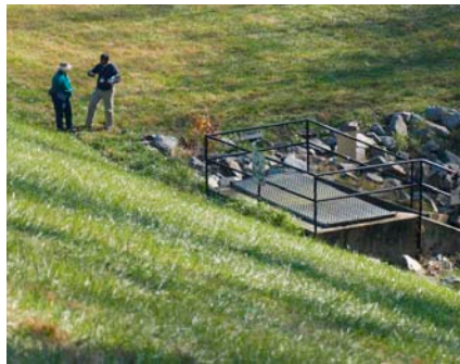
Back slope of Pohick Site 2 dam.
