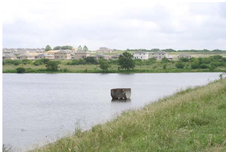
Plum Creek Dam No. 5 was built in a rural area that has become urbanized in recent years.
