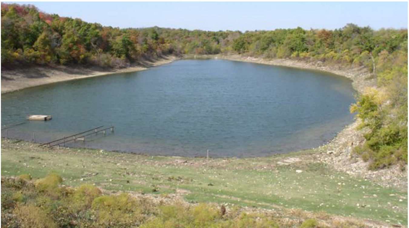
Upper Clear Boggy Watershed Dam No. 35 is part of a 113,482-acre watershed.
