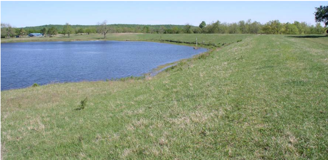
Upper Clear Boggy Watershed Dam No. 34 is part of a 113,482-acre watershed.
