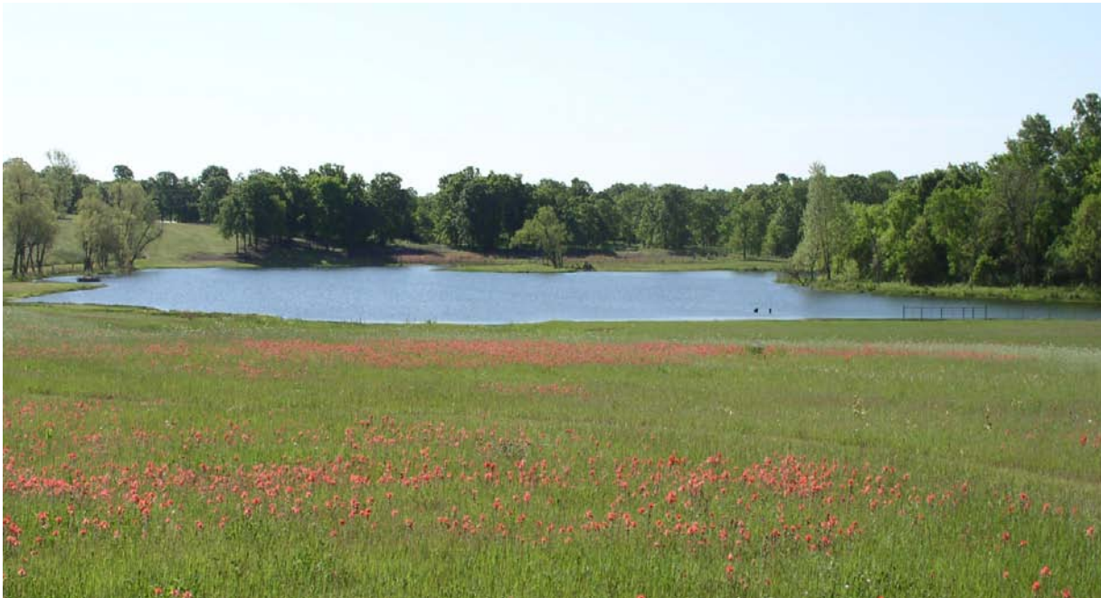
Upper Clear Boggy Watershed Dam No. 33 is part of a 113,482-acre watershed.
