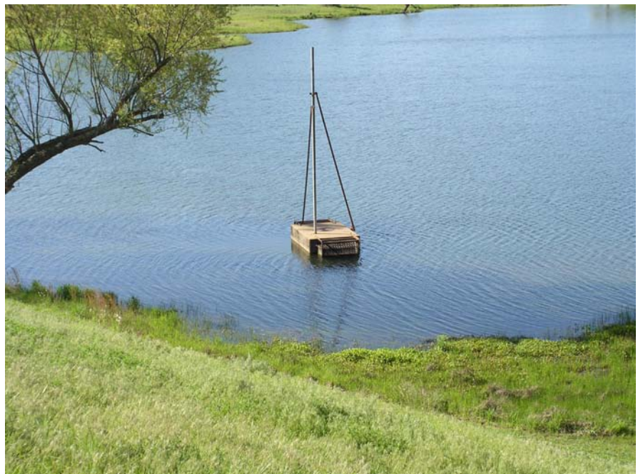
Existing principal spillway inlet on Upper Clear Boggy Watershed Dam No. 33.
