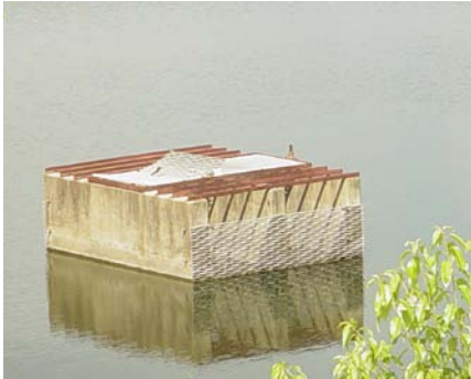
The principal spillway inlet tower at Sallisaw Creek dam.
