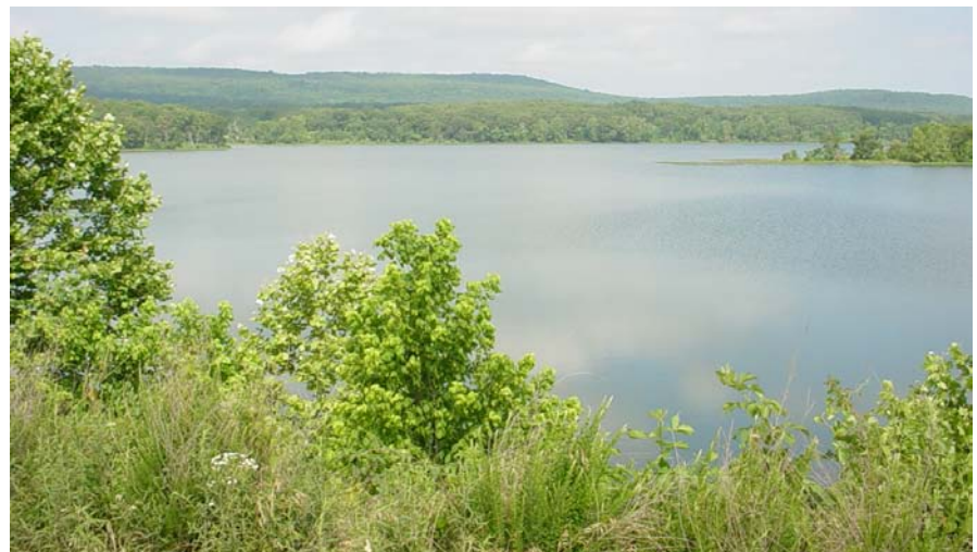
The dam provides 3,000 acre-feet of municipal water storage.
