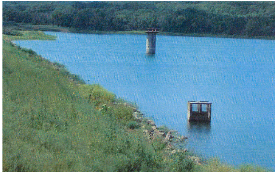
Sallisaw Creek Watershed Dam No. 18M protects the City of Stilwell from floods and provides water for 20,000 people.
