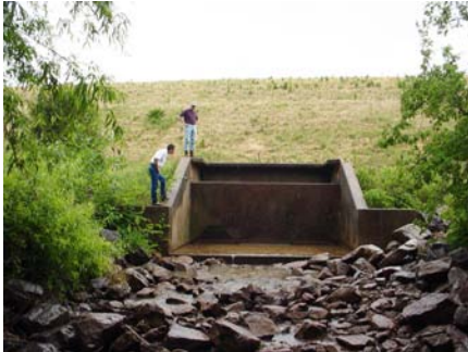
The outlet structure at Cottonwood Creek dam.
