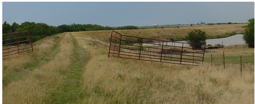
The existing dam at Cottonwood Creek Watershed.
