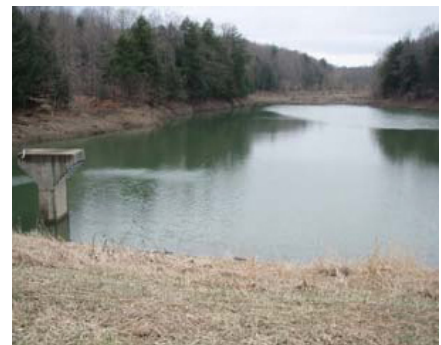
View of the flood retaining pool and riser on Conewango site 3 from the top of the dam. The dam will be raised to meet modern safety criteria.
