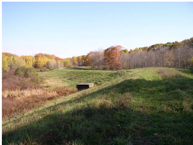
The Hop Brook Dam in Northborough, Massachusetts provides flood protection and recreational benefits.
