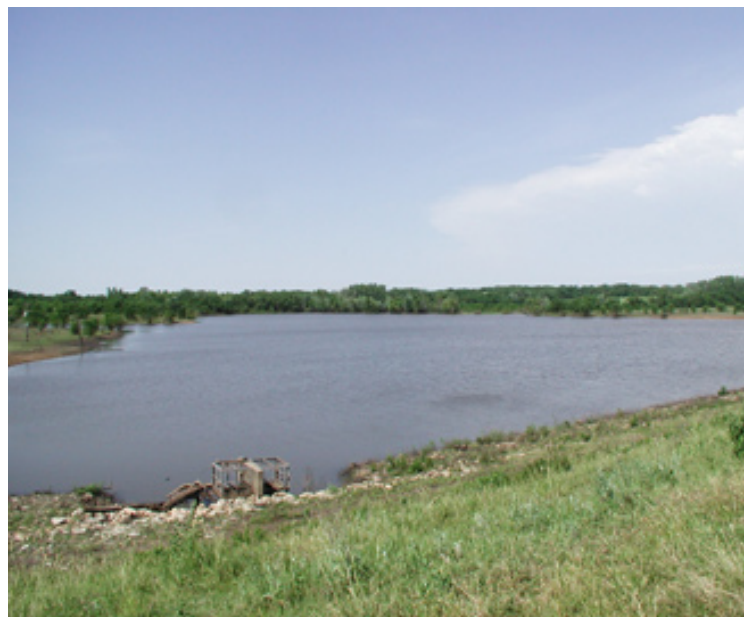
The watershed project is a high hazard class dam which protects the east part of the city of Burlingame, Kansas from flooding.
