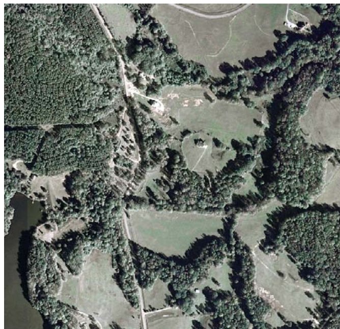
Aerial view of the South River Dam No. 4 site.
