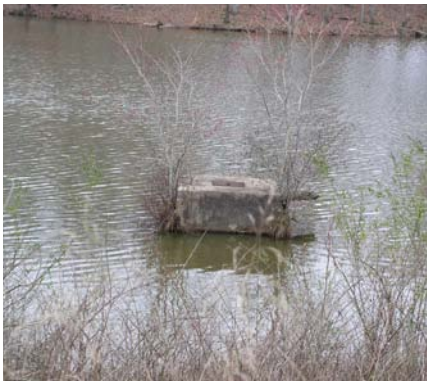
South River Dam No. 4. Principal spillway inlet.
