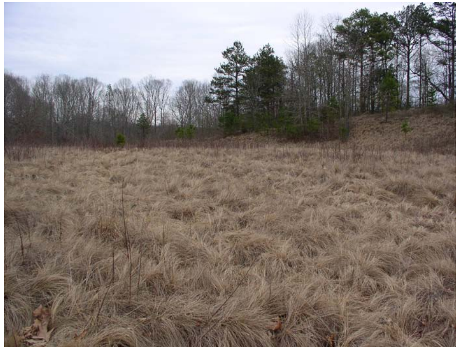
South River Dam No. 4. Well vegetated auxiliary spillway.
