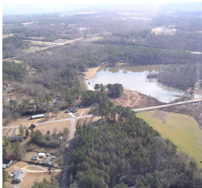
Aerial view of the Marbury Creek Dam site.
