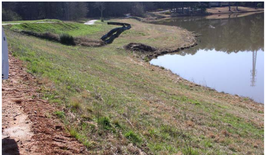
Marbury Creek Dam 22. Maintenance performed on east end of dam.
