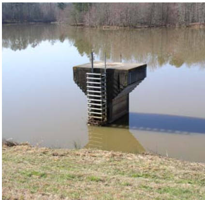
Marbury Creek Dam 22. Principal spillway inlet structure.
