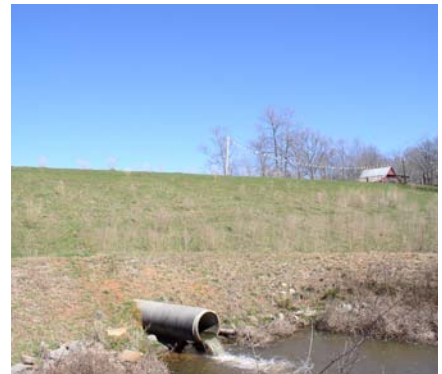
Little Sandy Trail Creek Dam 1. Principal spillway outlet.
