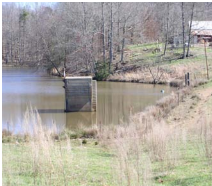
Little Sandy Trail Creek Dam 1. Principal spillway inlet.
