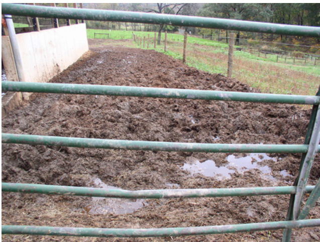
Before animal walkway was installed.
