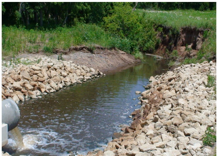
Plunge basin spillway outlet on Upper Red Rock Watershed Dam No. 52.
