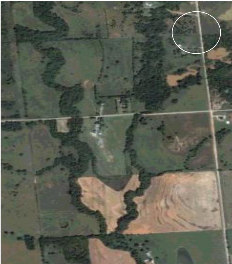
Aerial view during the construction of the dam shows homes, agricultural land, and roads downstream of Stillwater Creek Watershed Dam No. 33C.
