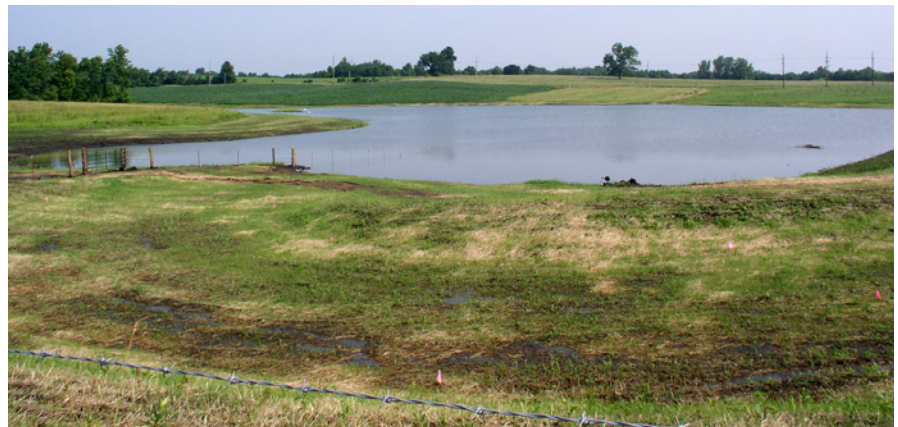
This single purpose floodwater retarding dam is one of 112 structures that have been completed in the Big Creek-Hurricane Creek Watershed. The pool of this structure measured 2 feet deep after a heavy rain. The spillway safely releases stormwater after significant storm events.
