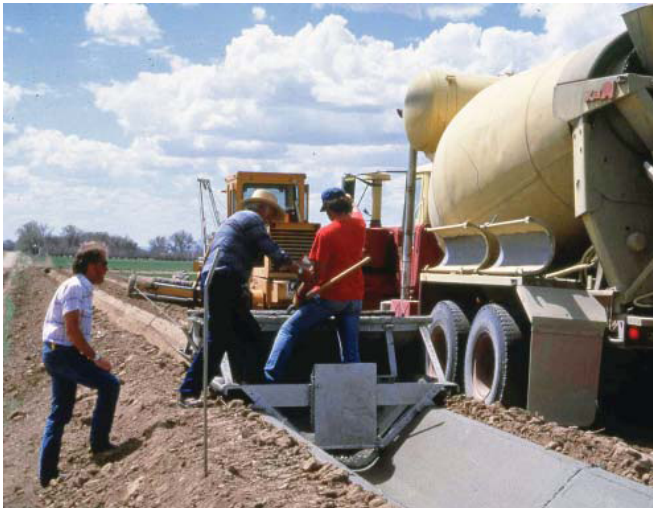
Installation of concrete ditch to conserve water.
