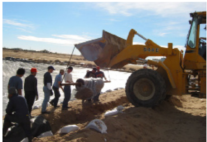
Placement of final piece of liner.
