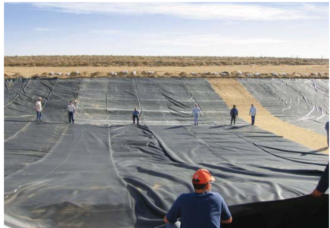
Installation of lining.
