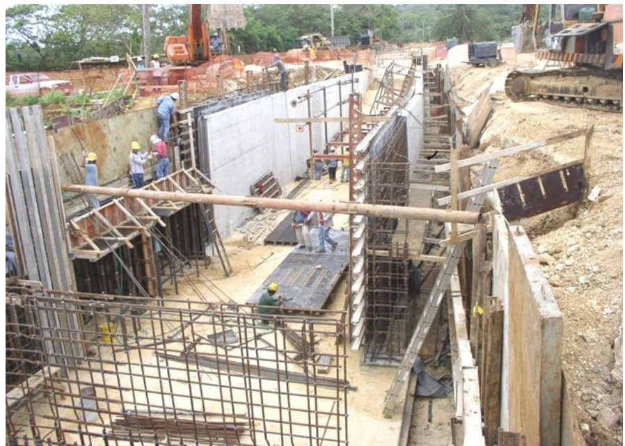
Previous construction phase.
