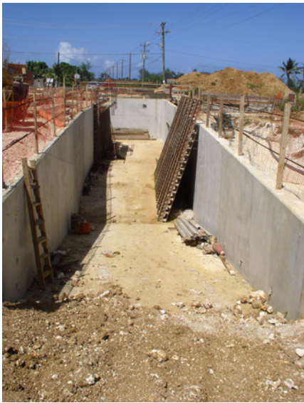
Previous construction phase.
