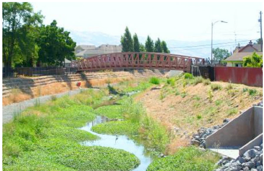
In Reach 3, an already completed section of the project, trapezoidal concrete was replaced with multi-benefit designs combining flood control, habitat, and community parks and bridges.
