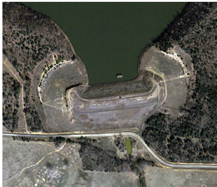
An aerial view of Site 9 of the Upper Petit Jean Watershed dam west of Booneville, Arkansas.
