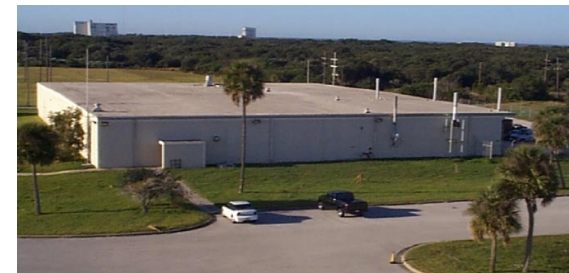
Figure 5. Engineering Support Building at NASA’s Launch Complex 34, where an innovative nanotechnology solution was implemented to treat chlorinated solvents in groundwater
